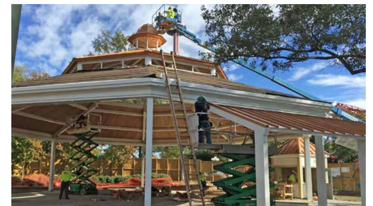
Installation of metal roofing panels
