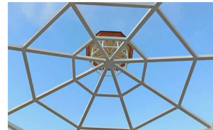
Frame complete and ready for roofing
