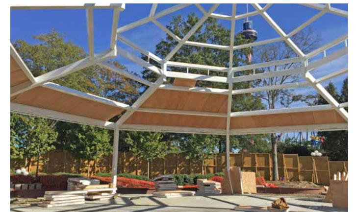
Supporting roof deck is installed
