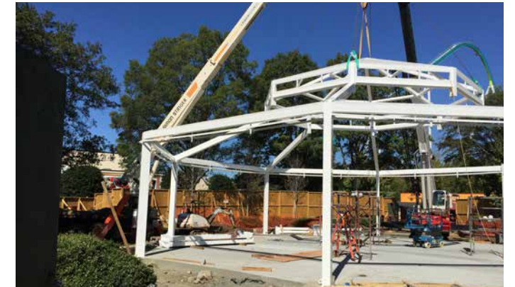
No field welding required during erection
