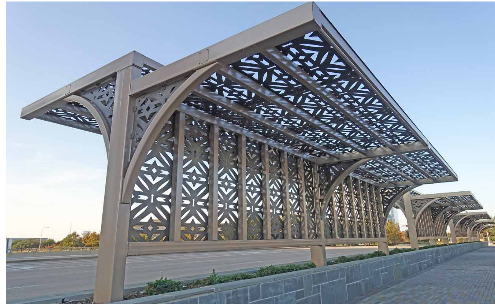
Cantilevered Walkway Cover 18x34 w/ laser-cut panels #62566
