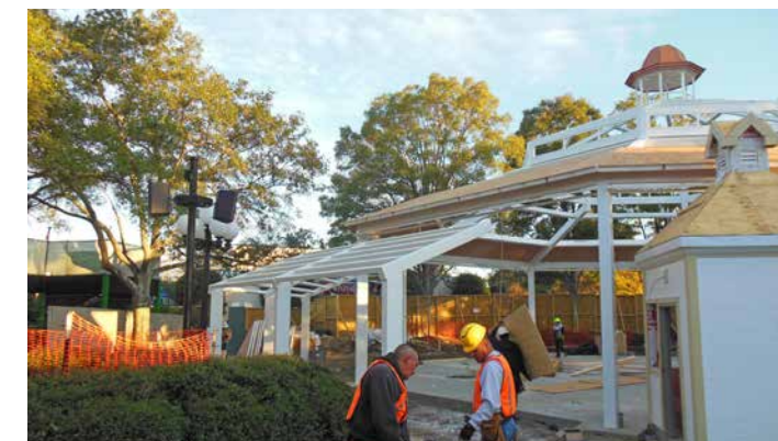
Installation of metal roofing panels
